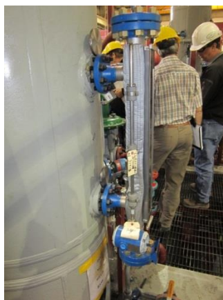
Revision 3 Studding Outlets with Site Glass
