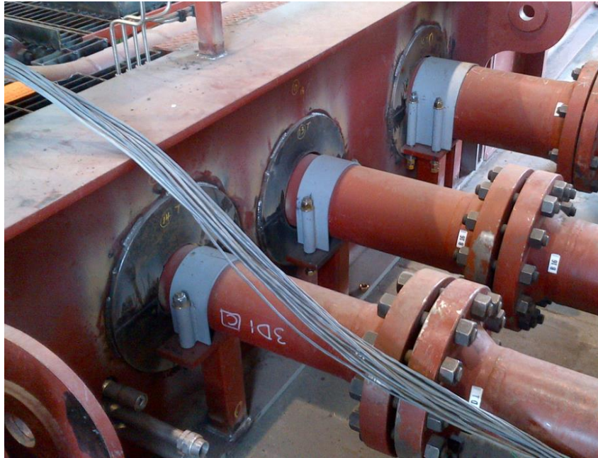
Figure 23: Pipe Clamps for Vibratory Service
