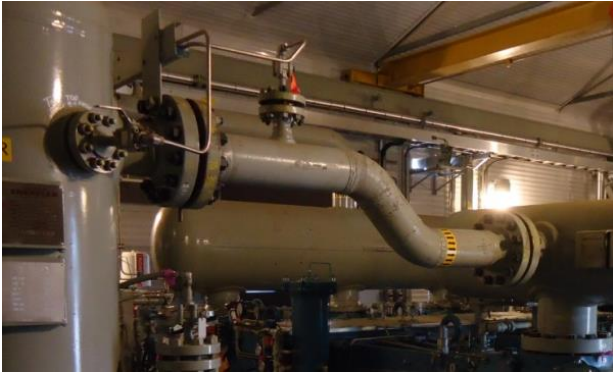
Revision 1: Conventional Connection Tee
