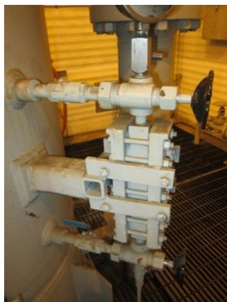
Revision 1 and 2 Conventional Site Glass Attachment
