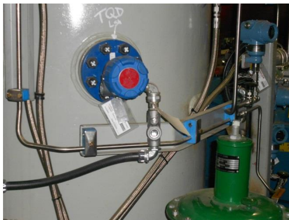
Revision 4 Site Glass Replaced with Ultrasonic Level Switches
