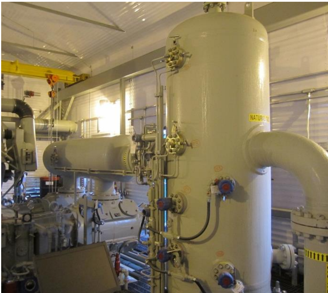
Figure 15: Robust Small-Bore Attachment Design at Sundance is the Result of Continuous Improvement and Effective End-User Specification.
