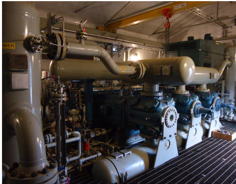
Figure 21: Plate-Type Outboard Cylinder Supports
