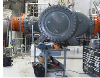
Troubleshooting support at gas pipeline facility
