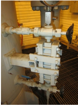
Revision 1 and 2 Conventional Site Glass Attachment
