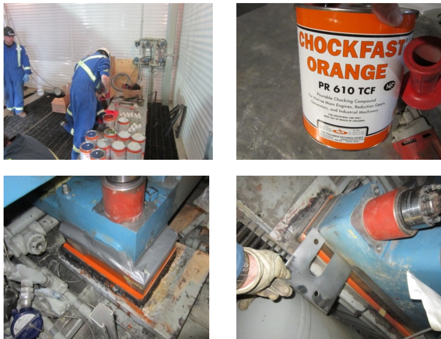
Figure 11: Grout Box Mount
