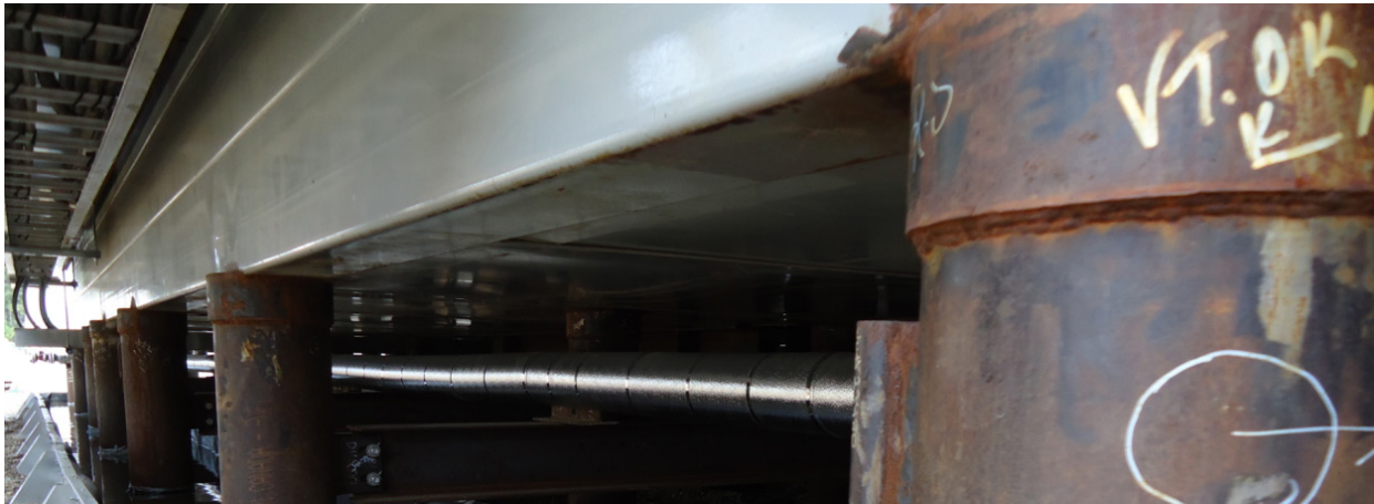
Figure 3: Piles Attached to Skid with slip-rings for Saturn 1, 6500 HP KBZ/6 compressor package
