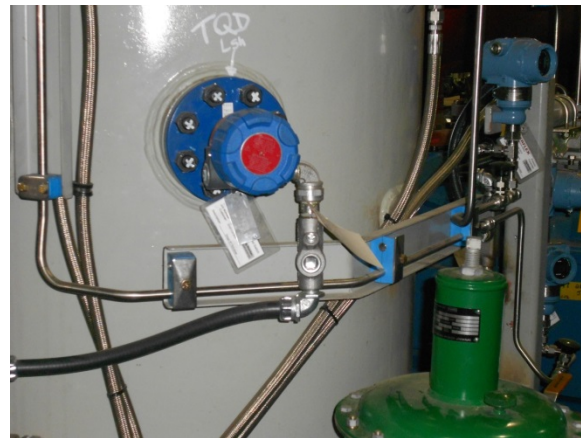
Revision 4 Site Glass Replaced with Ultrasonic Level Switches
