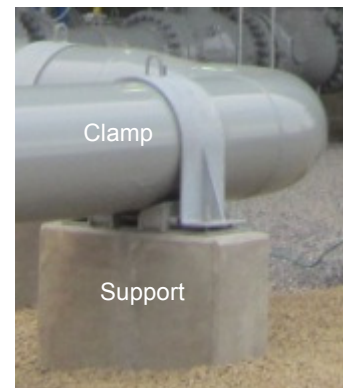
Figure 2. One-gusset type clamp with wedge blocks and concrete pier support
