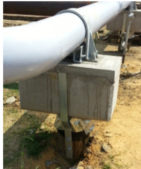
Figure 4. Poor support design
