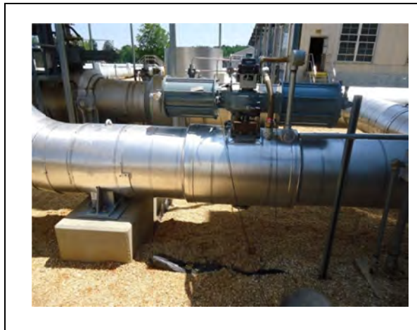
Figure 2. Unit 16 Surge Valve Operator
