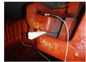
Testing effectiveness of temporary winding supports
